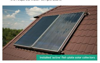
Flat plate or evacuated tube? A flat-plate system
