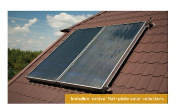
Flat plate or evacuated tube? A flat-plate system
